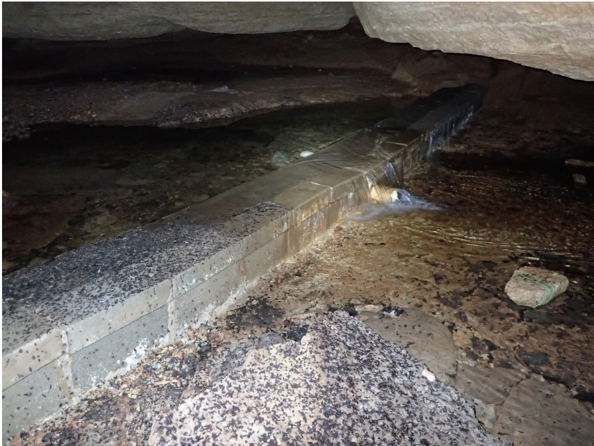
Figure 3. Barrier installed in Tumbling Creek to stop movement of gapped ringed crayfish Faxonius neglectus chaenodactylus to upstream reaches of the cave. Total height of the barrier is 29 cm and the top 9.5 cm of this wall overhangs the bottom portion on the downstream side by 2.5 cm. Since the barrier was completed, only a few crayfish have been found and removed from above the barrier (not as part of a biological survey)
