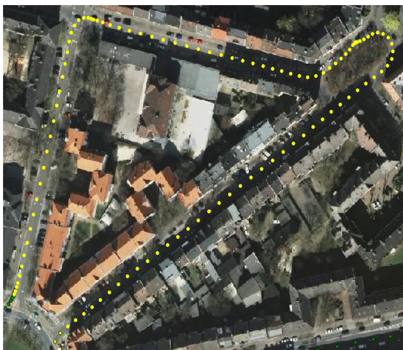
Figure 7. Path segment with close buildings and trees.
