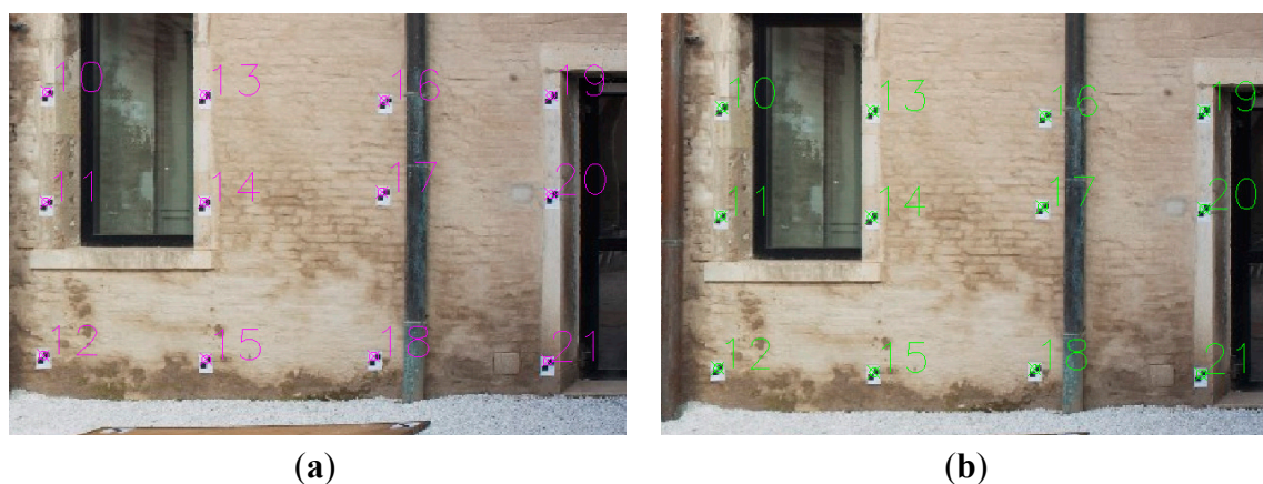
Figure 18. The rectification of the original (a) and undistorted NIKON D100 images; (b) lead to an RMS error of the collected GCPs of 0.0013 m and 0.0001 m using the VeCAD-Photogrammetry application [20].
