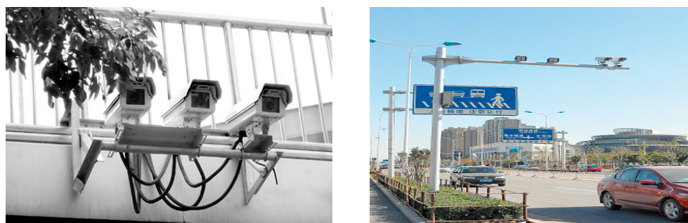
Figure 2. Multi-cameras road monitoring systems.
