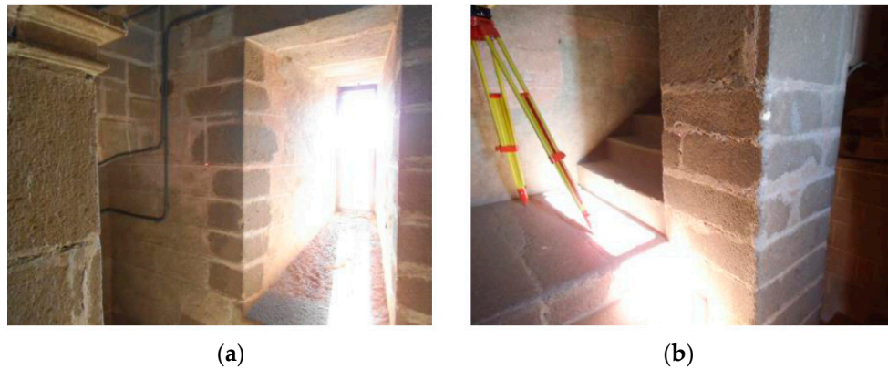
Figure 10. Walls built with granite ashlars (a,b). Interior of Santa María Church, Guareña (Spain).
