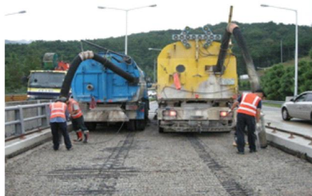
Figure 11. Bridge overlay site.
