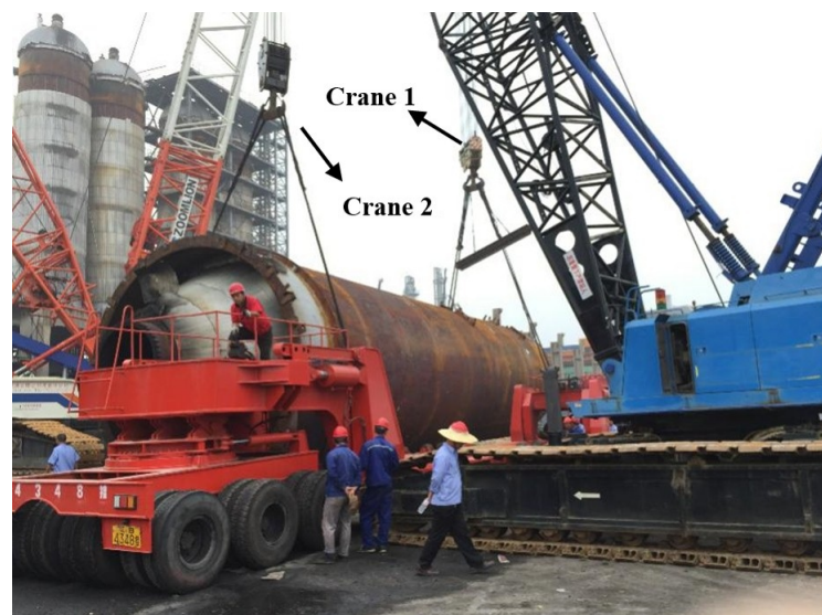
Figure 5. The hoisting work process.
