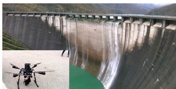
Figure 2. Ridracoli dam while overflowing. Small panel: HIGHONE 4HSEPRO quadrotor mounting a gimbal system and a SONY Alpha 7R while at rest.
