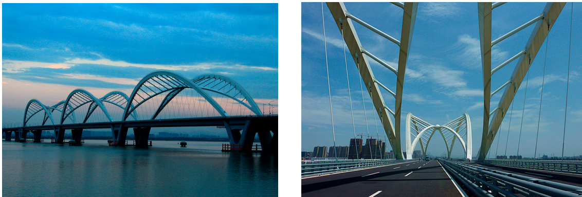
Figure 3. Overview of the Jiubao Bridge.
