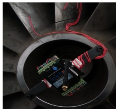
Figure 19. The installation of wireless strain node.
