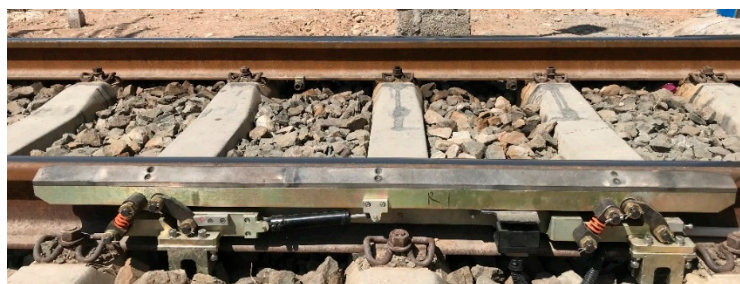
Figure 15. The photo of the installed parallelogram mechanism.
