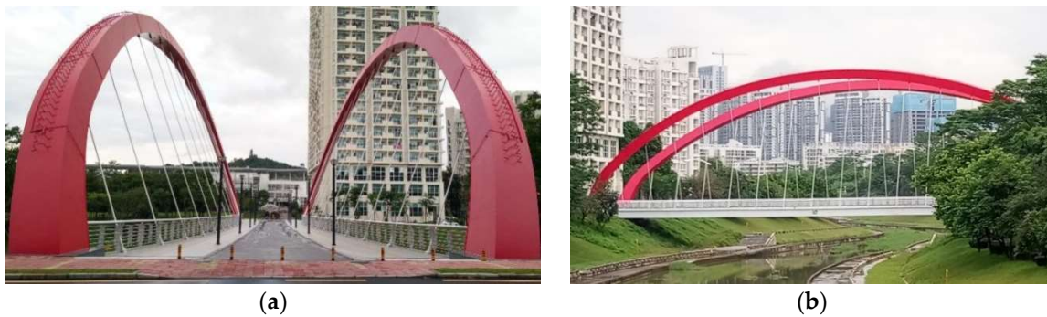
Figure 6. Front view and lateral view of the Rainbow Bridge: (a) front view; (b) lateral view.
