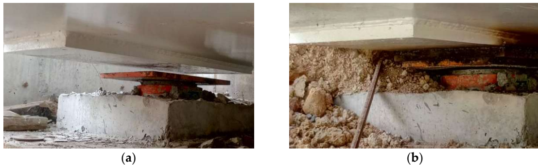
Figure 16. The change of the boundary condition: (a) before the 17th day (5 April 2017); (b) after the 17th day (5 April 2017).
