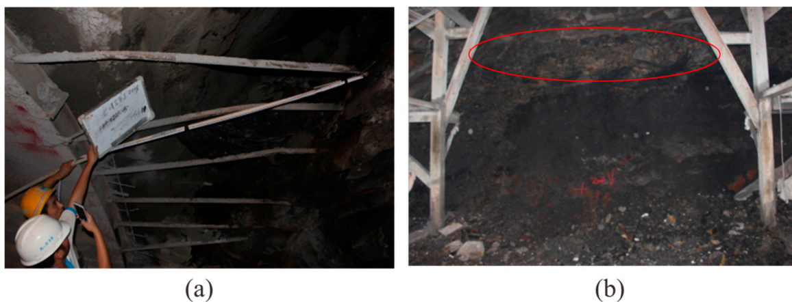
Figure 16. Tunnel face at (a) K3 + 024.5 and (b) K3 + 021.
