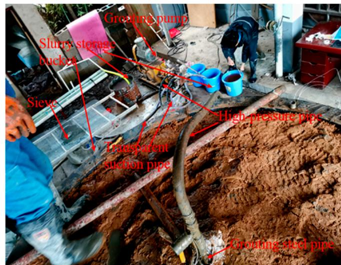
Figure 4. Grouting system equipment.
