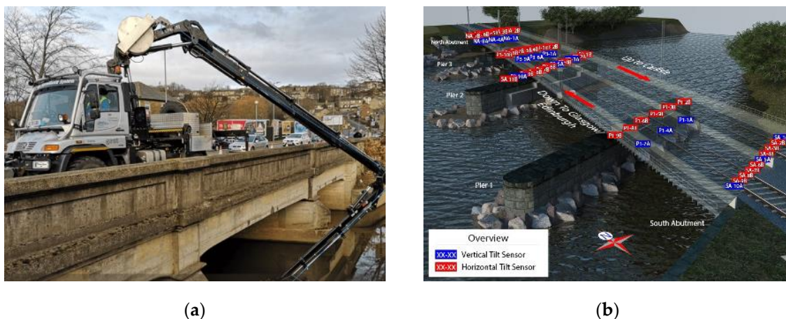
Figure 2. (a) BridgeCat technology for bridge inspection [40]; (b) Layout of the Structural Health Monitoring (SHM) system installed at the Lamington viaduct (courtesy of Network Rail).
