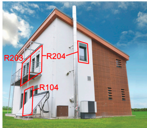
Figure 1. The wooden building of the passive standard located in the Faculty of Civil Engineering, VSB—TU Ostrava with selected smart home (SH) rooms R204, R203, and R104 [15].
