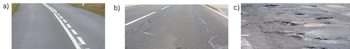
Figure 2. The example of the road surface classified in the paper as: (a) A good, (b) B slightly damaged, (c) C bad.
