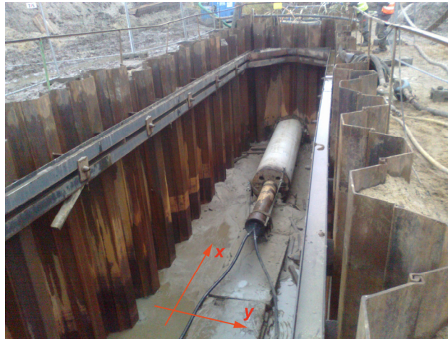
Figure 1. Impact installation of a pipe segment.
