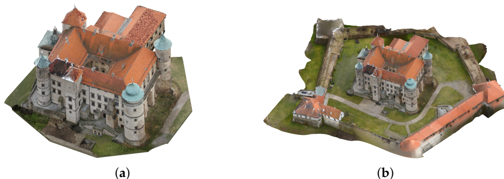
Figure 12. Polygonal models of the castle in Nowy Wiśnicz: (a) building only (4,133,352 faces), (b) the building with fortifications (1,966,487 faces).
