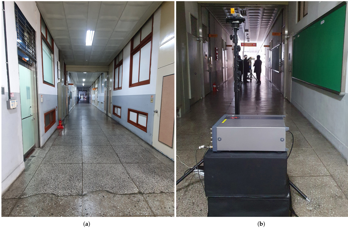
Figure 5. (a) The figure shows the 375 m-long corridor without human movement on the 3rd floor of the main building just before the measurement campaign; and (b) it shows a measurement scenario of the 3rd floor corridor of the main building.
