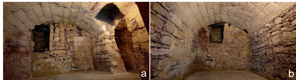
Figure 9. Underground rooms: (a) the sepulchral cell VI; (b) the sepulchral cell VII.
