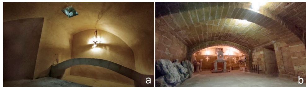
Figure 11. Underground rooms: (a) the cistern (IX); (b) the food warehouse (XI).
