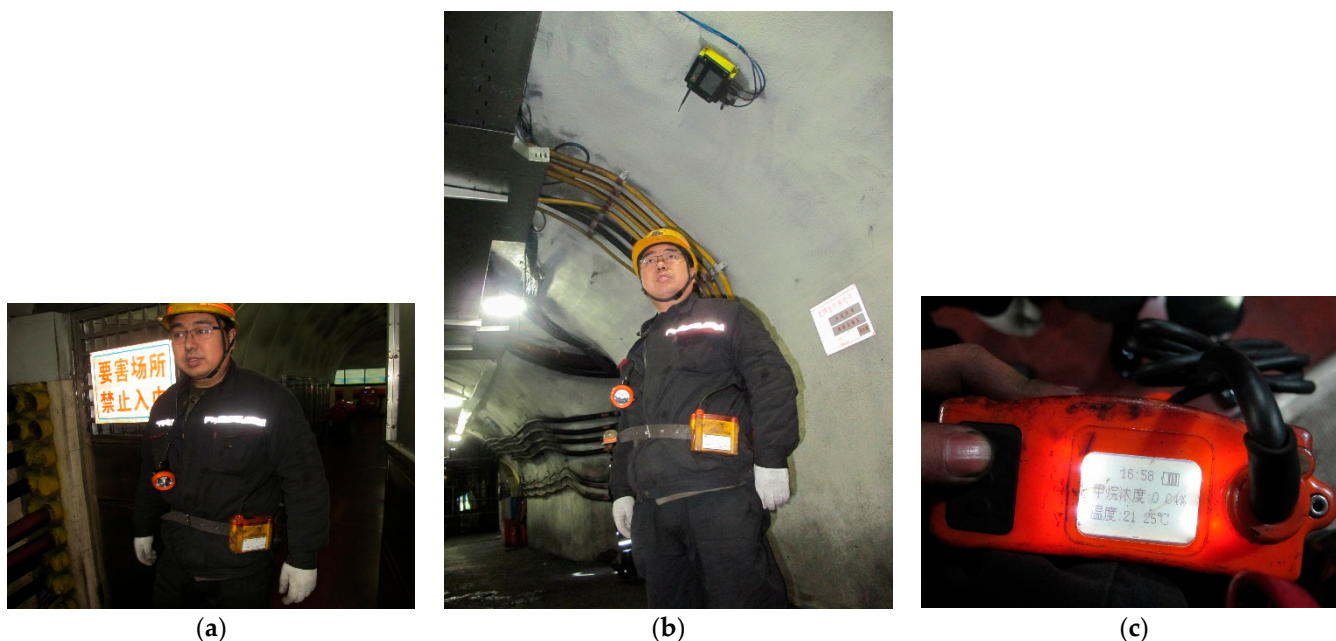
Figure 3. Network model of monitoring system. (a) Miner and smart miner’s lamp, (b) fixed gas sensor and wireless access point, (c) gas monitoring data.
