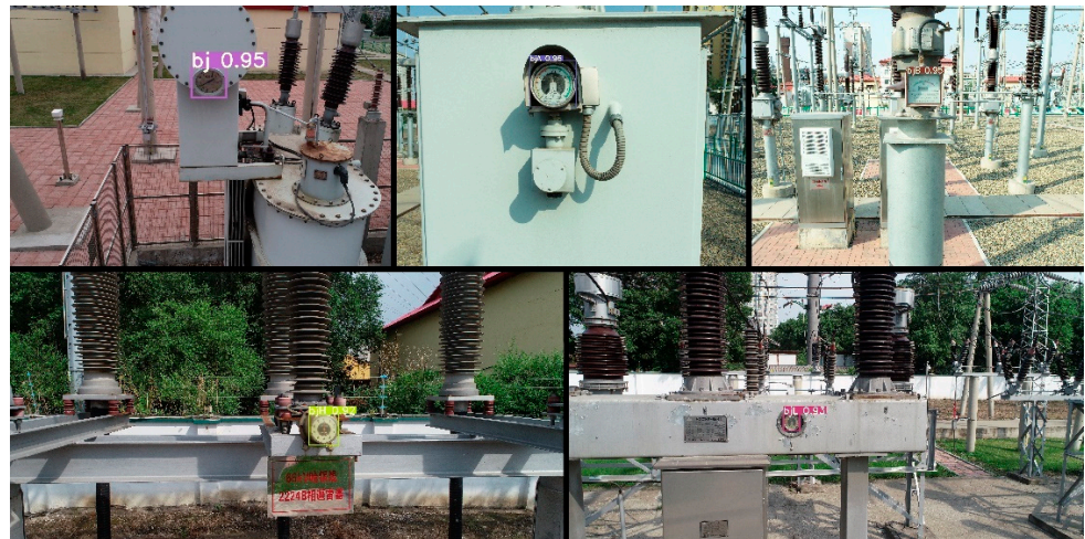
Figure 6. Dial detection results using YOLOv5s.
