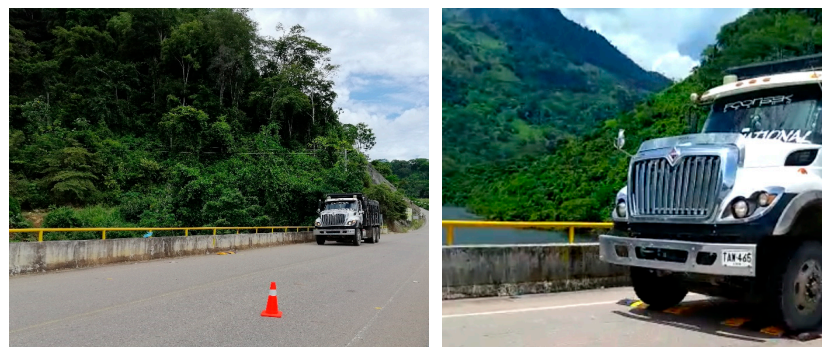
Figure 14. Three-axle 32-ton truck moving at a speed of 40 km/h on the Tablazo bridge.
