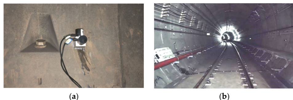
Figure 21. Field test diagram. (a) Acceleration measuring point of tunnel wall. (b) Overall view.
