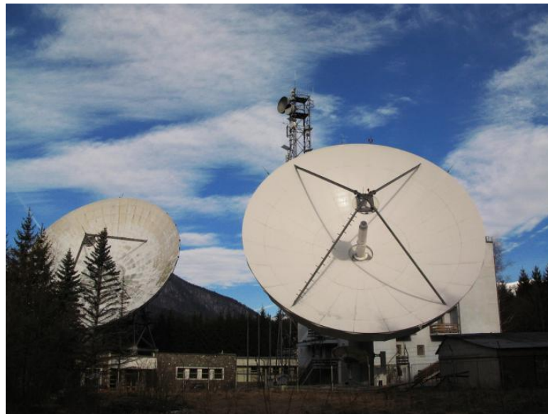
Figure 3. The two antennas at Cheia Satellite Communications Center.
