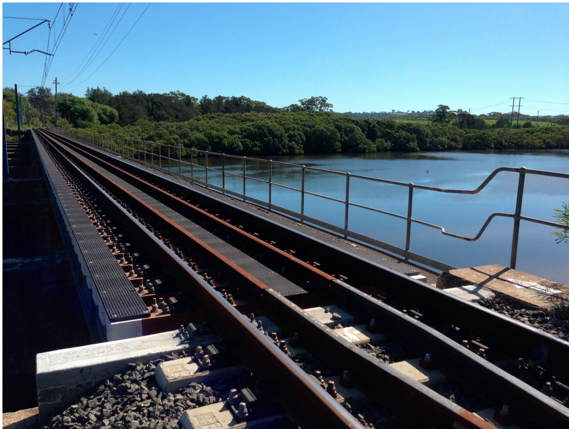
Figure 1. The Minnamurra Railway Bridge in New South Wales, Australia.
