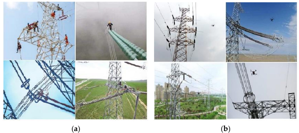
Figure 1. Insulator inspection. (a) Manual inspection. (b) UAV inspection.
