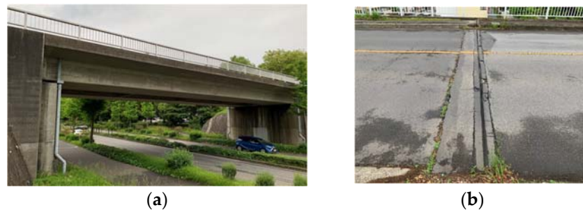
Figure 5. The view of the bridge: (a) full view; (b) expansion joint [48].
