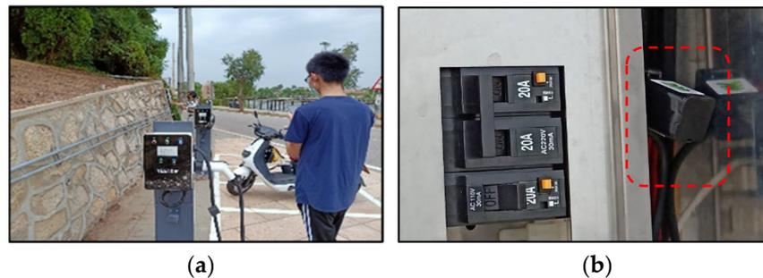
**Figure 11.** (a) Field picture with charging piles, (b) power distribution box with an IoT clamp-meter marked in red.
