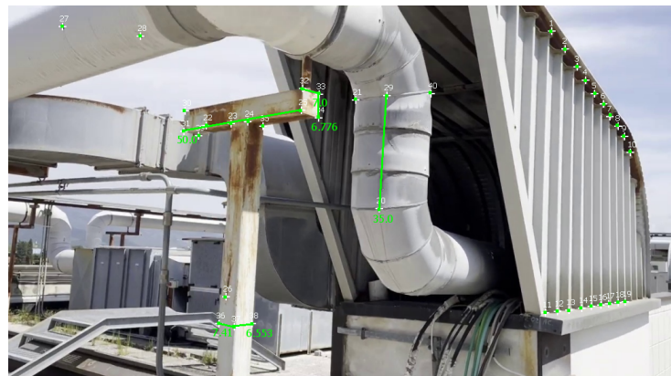
Figure 16. Measurements computed in MoReLab. The distances of 50, 35, and 7 cm are provided for calibration, and other distances are calculated.
