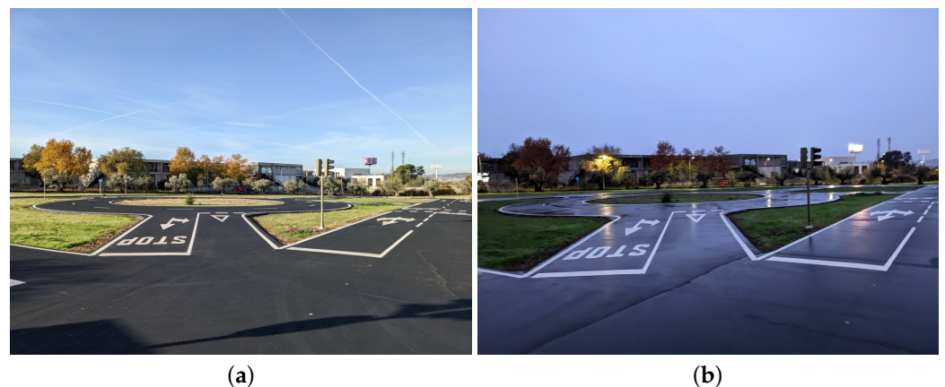
Figure 1. RGB view of a roundabout entrance. (a) Day view in dry conditions. (b) Night view in wet conditions.
