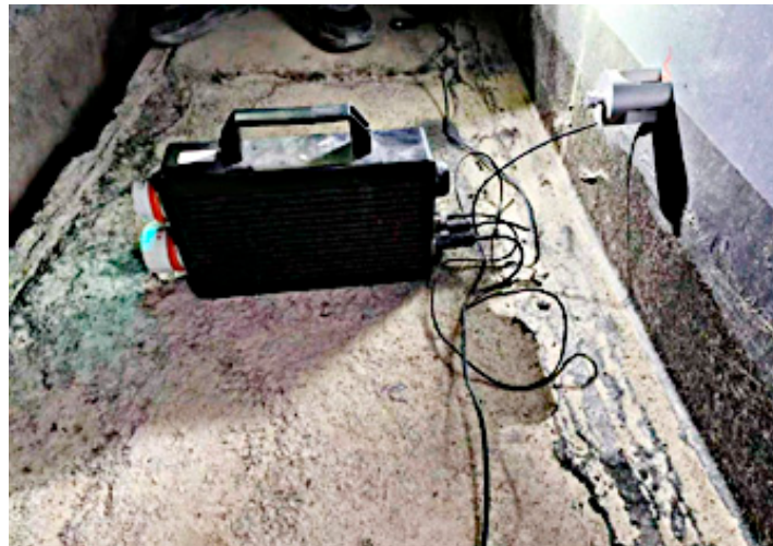
Figure 6. On-site installation of a piezoelectric ceramic sensor.
