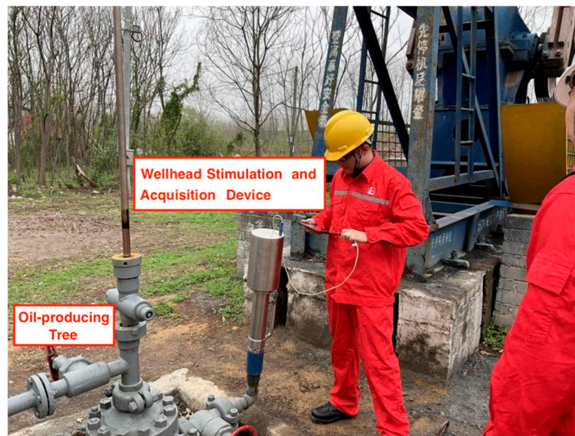
Figure 24. Wellhead detection device and on-site installation at the oilfield.
