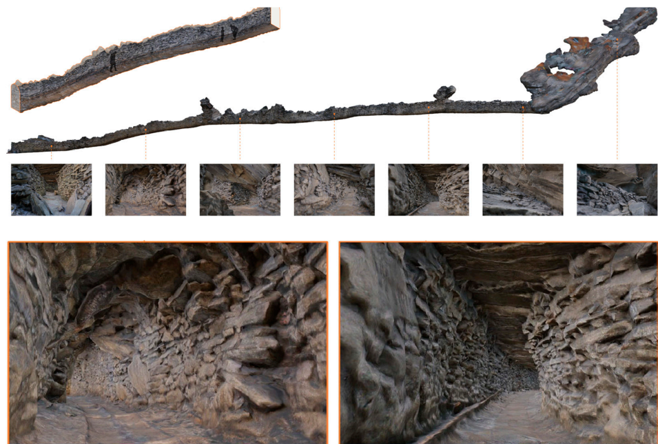
Figure 23. The 3D model generated from an Ant3D survey of an abandoned mining tunnel. Images extracted from a prior publication; additional details on the processing can be found at [24].
