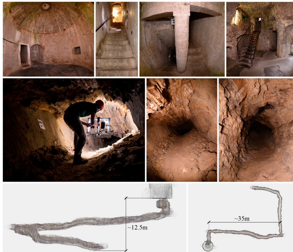
Figure 1. Some images of the San Vigilio Castle's tower ( top ) and tunnel ( centre ); and the dimensions of the tunnel ( bottom ). The image refers to the FINE benchmark dataset.
