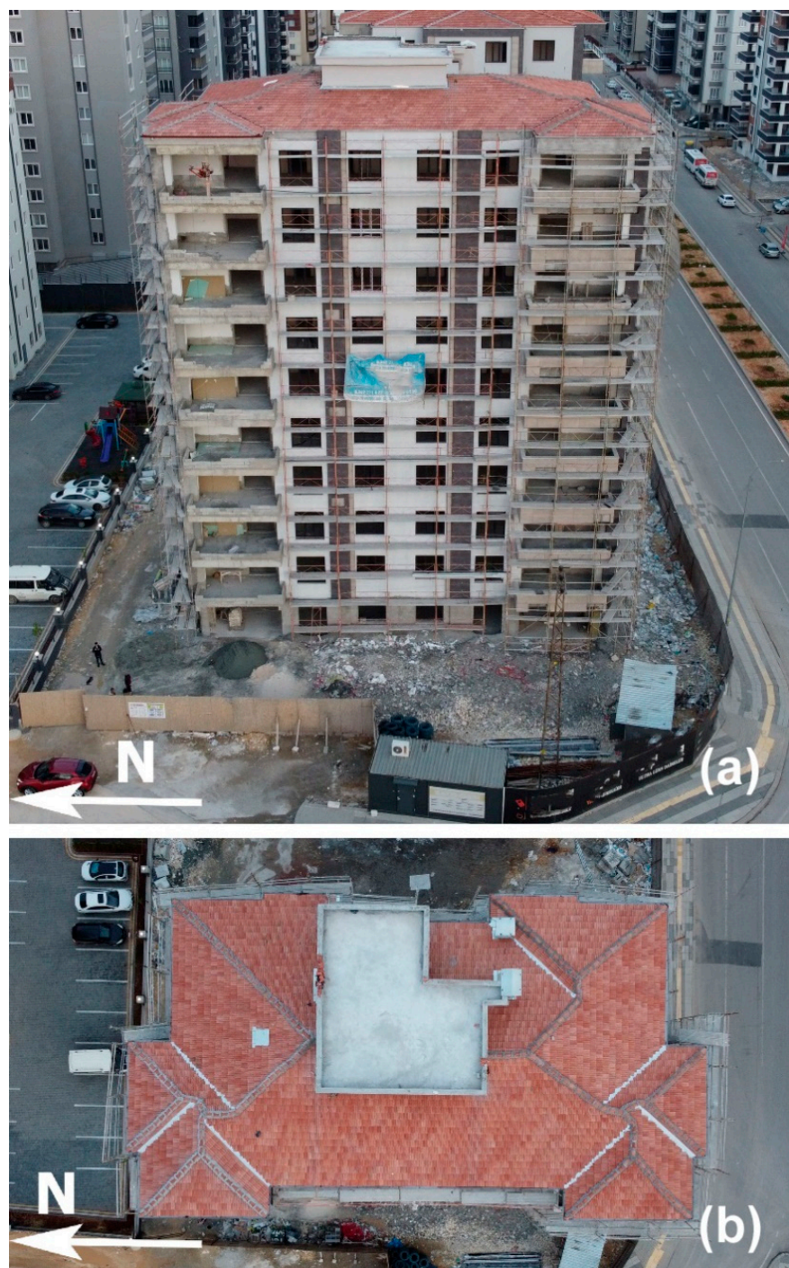
Figure 16. Aerial photos of the building from (a) side and (b) top.
