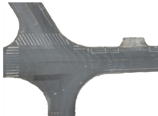
Figure 20. Result of road reconstruction.
