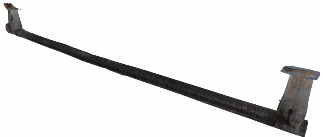
Figure 26. Textured 3D model of the drainage pipe based on bidirectional data.
