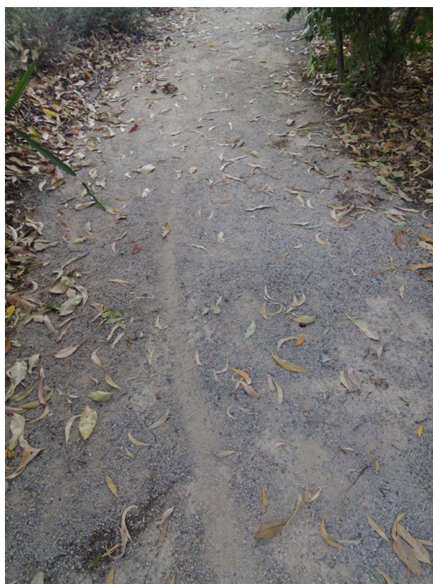
Figure 5. Loose gravel path.
