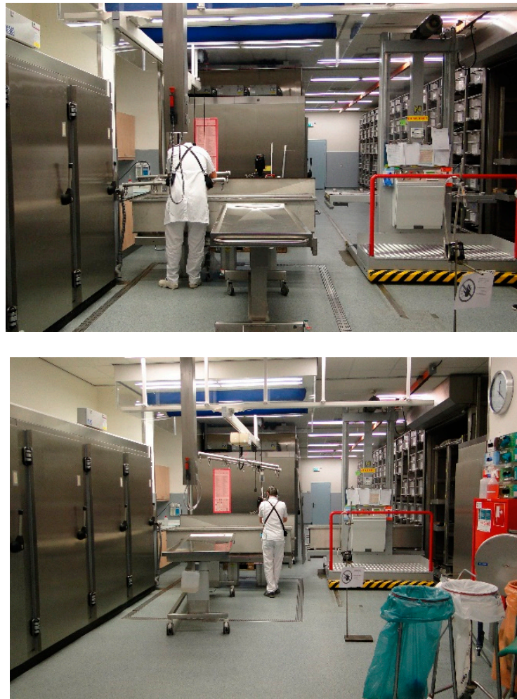
Figure 7. Take-out preparation from storage tank ( upper panel ) and place back preparation in storage tank ( lower panel ) (O-1 in Table 2).
