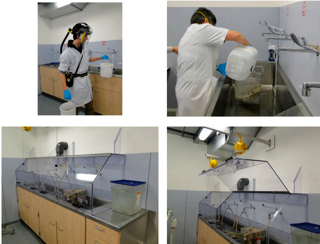
Figure 5. Before (upper panels) and after (lower panels) introduction of a Perspex cover with local exhaust ventilation (T-3 in Table 2).
