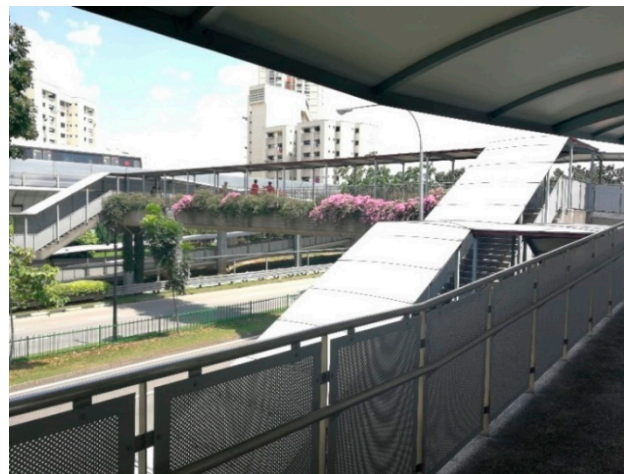
Figure 6. An overhead bridge with stairs and long ramps.
