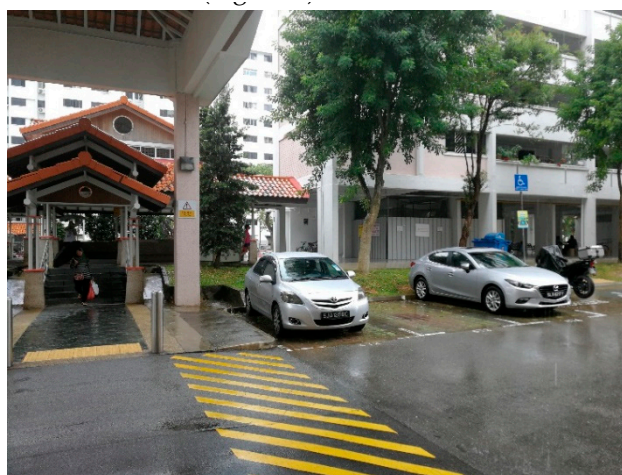
Figure 7. Sheltered stairs with an unsheltered slope nearby.
