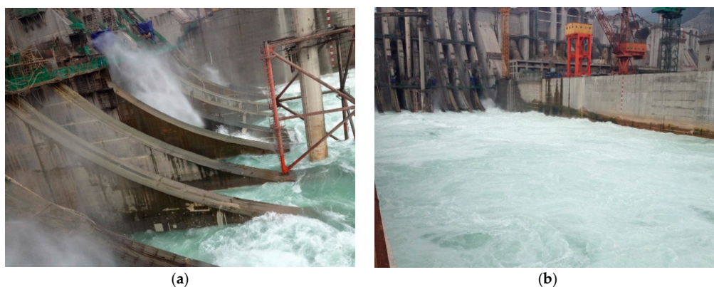
Figure 18. Photographs of the flow discharge operation of the XHS. (a) Flow pattern of orifice flow. (b) Flow pattern in plunge pool.
