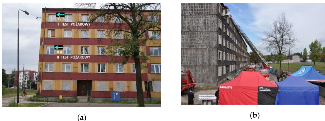
Figure 1. Pictures of a residential building at Poczтовая Str. 15 in Bytom from the north, scheduled for fire tests: (a) before the removal of facade panels containing asbestos (July 2012); (b) on the day of the experiment (20 September 2012).
