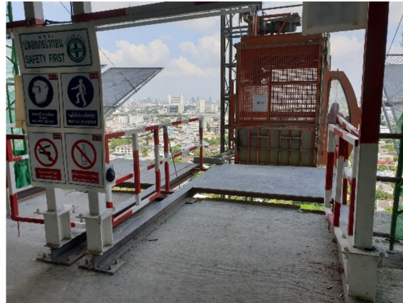
Figure 4. Landing platforms for hoist lift.
