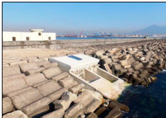
Figure 9. Lateral view of the OBREC device in Italy (Reprinted from Sustainability, Contestabile et al., 2016).
