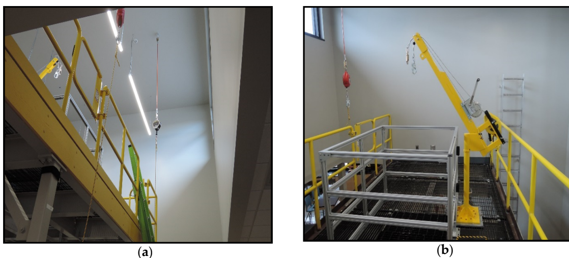
Figure 2. Personal fall arrest anchorages: (a) ceiling mounted anchor, (b) davit on the mezzanine.
