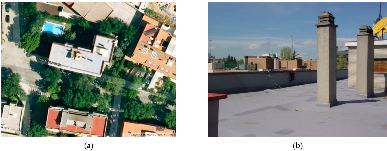
Figure 1. (a) Aerial photograph of the building in Madrid; (b) detail of the building roof.
