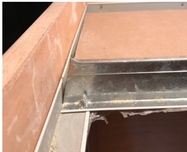
Figure 15. Intersection of frame and trim after cutting.
