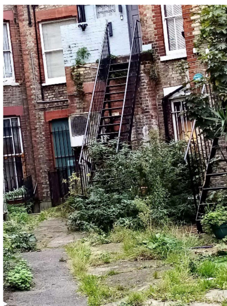
Figure 23. “The staircase leading into my apartment.”—Participant.Survey15.
