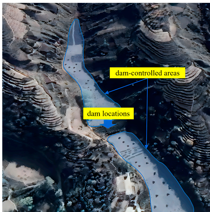
Figure 1. Check dam system in the Yellow River Basin.
